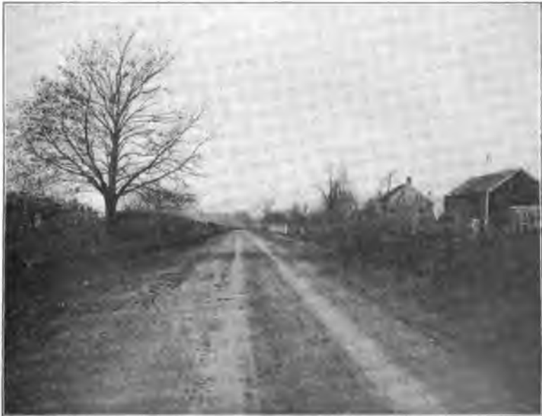
Neshanic road, Somerset Co., after improvement.
